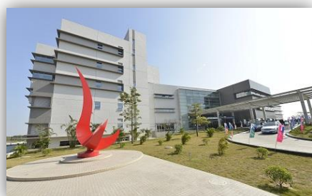
New FYTRI Building at Nansha IT Park, opened in December 2014
